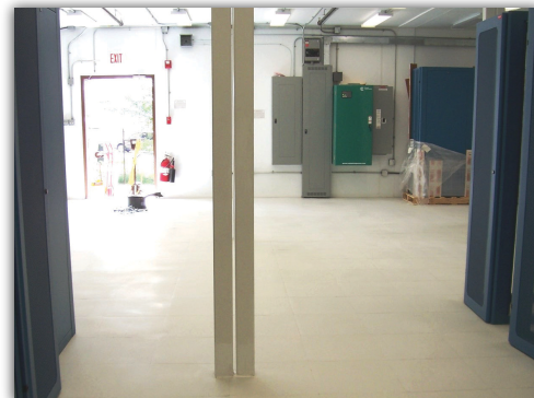
FreeStyle™ CVT provides industry-leading static protection in this server room application.
