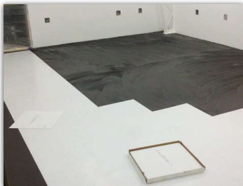
FreeStyle™ CVT being installed in a server room, using trowel-on, 1-part, conductive adhesive.
