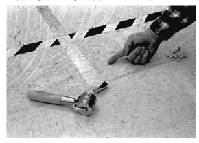
A thin coating of releasable adhesive should be applied on top of grounding strip to ensure good contact with carpet tile.
